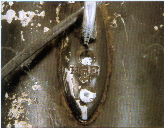
This marmite is marked with the initials of the manufacturer and the year when it was manufactured. The year could be shown in full or, as is the case here, by means of the last two digits. (G. Cano)
